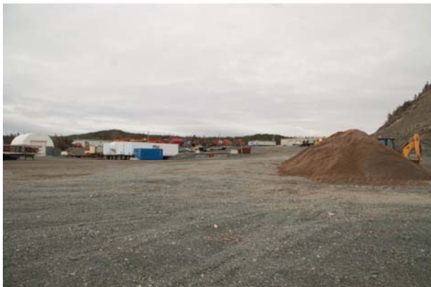
View of laydown area
