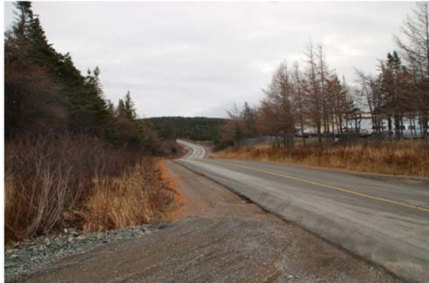
Looking northeast along Marine Drive
