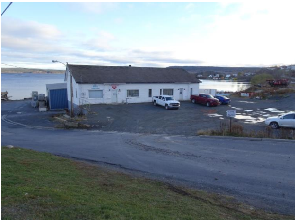
Office Exterior Office
