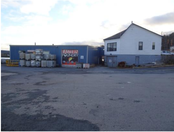
Foundry north elevation next to the office
