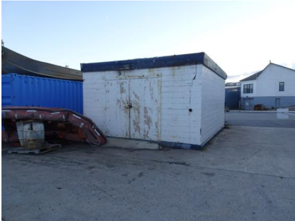
Welding Shop exterior north elevation
