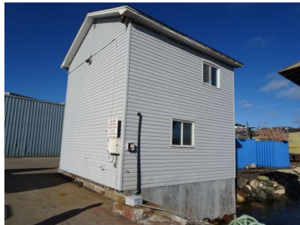
Wharf Office showing foundation
