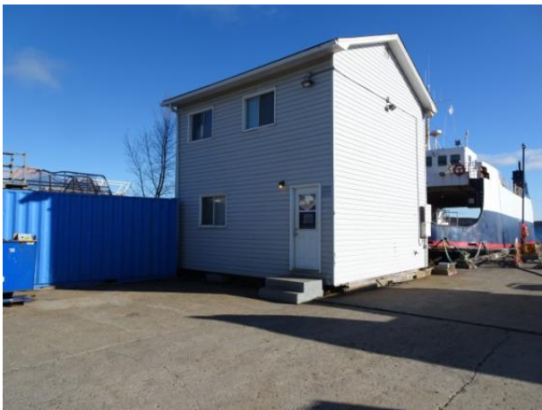
Wharf Office showing proximity to the finger pier
