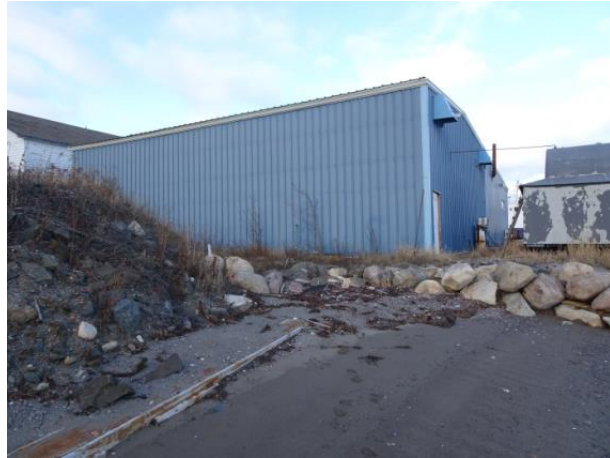
Foundry south and eastern elevations
