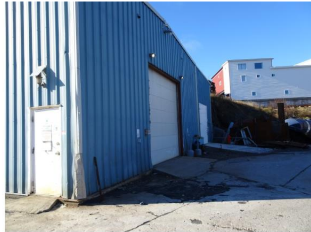
Machine Shop north elevation
